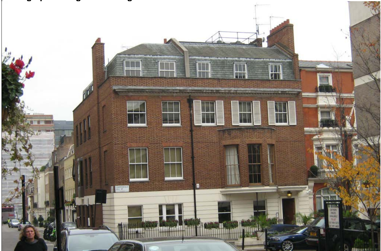
Photograph 1: Original building before demolition
